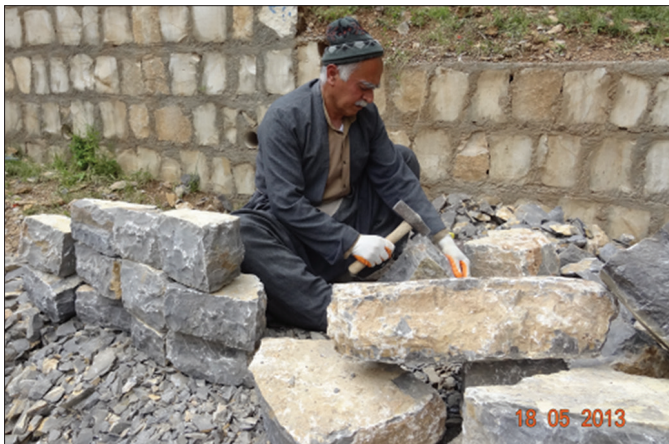
Fig. 2. Mason working on building site in town of Tewelle. (Author, 2013)
