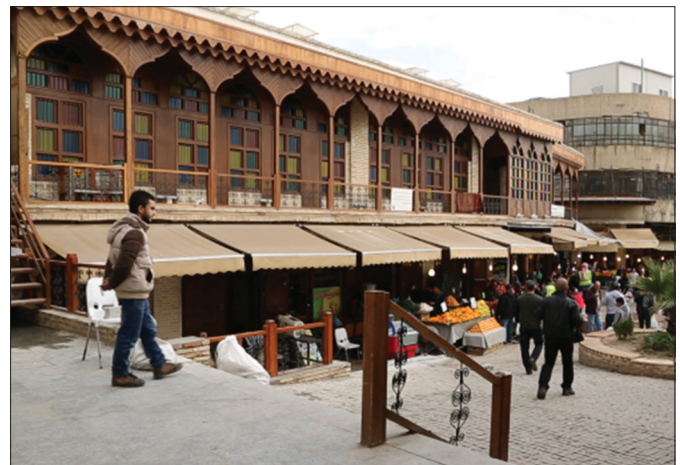
Fig. 22. Refurbished section of the entrance to the old bazaar. Site visit to city of Suleimani. (Author, 2015)
